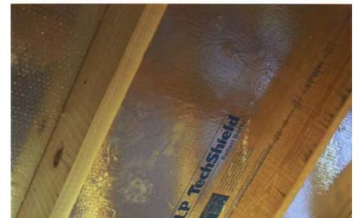
**Foil Barrier Insulation** for their metal building entry of a manufacturing facility for a sports lighting company using Super R Plus 97% Reflective Foil Radiant Barrier.
