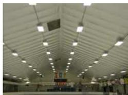
**Foil Barrier Insulation** for their metal building of an office/warehouse utilizing Tempshield Double Bubble two-sided Foil R-15 radiant barrier insulation.
