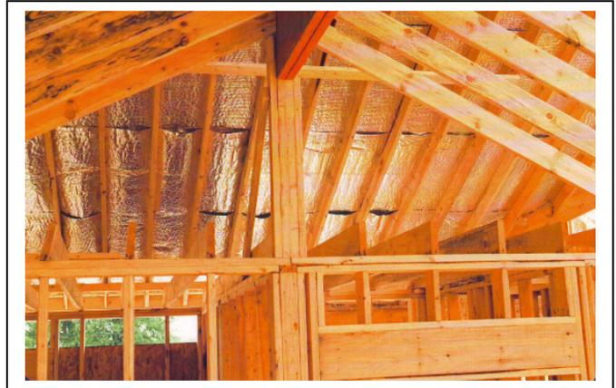
Cathedral ceiling - radiant barrier installed above the rafters, below the decking
