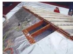
**Foil Barrier Insulation** for their residential entry utilizing Super R Plus Radiant Barrier Foil.
